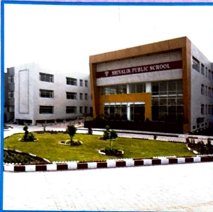
STATE OF THE ART INFRASTRUCTURE
